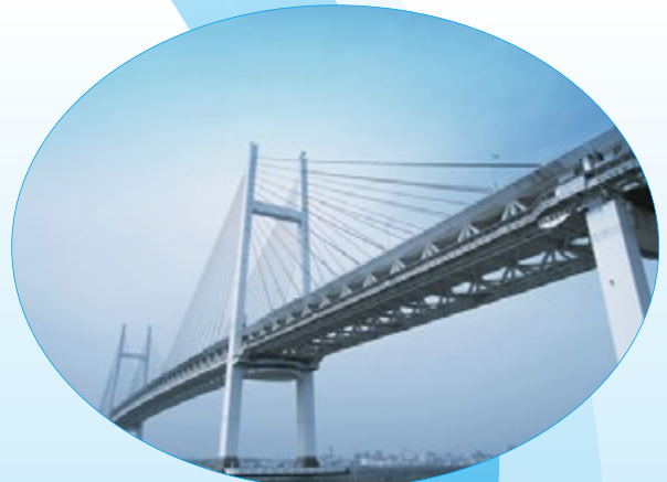
桥梁 Tower links & Cable hanger
